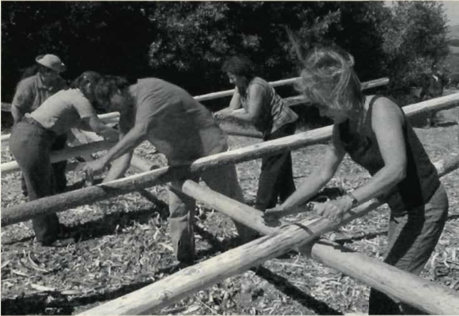
Stripping the Douglas Fir poles of their bark was a year-long project for Kule Loklo volunteers and PRNS staff. photo courtesy of Gordon Bainbridge
